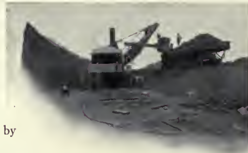
On Gatun Hill—A Steam shovel working in clay on the site of the locks.
