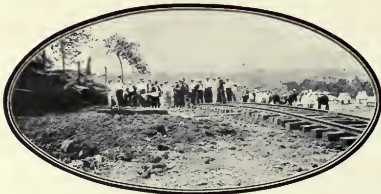
Site of the Gatun Dam — A view across the valley on the line of the proposed embankment 7,700 feet long and one-half mile thick at the base.
