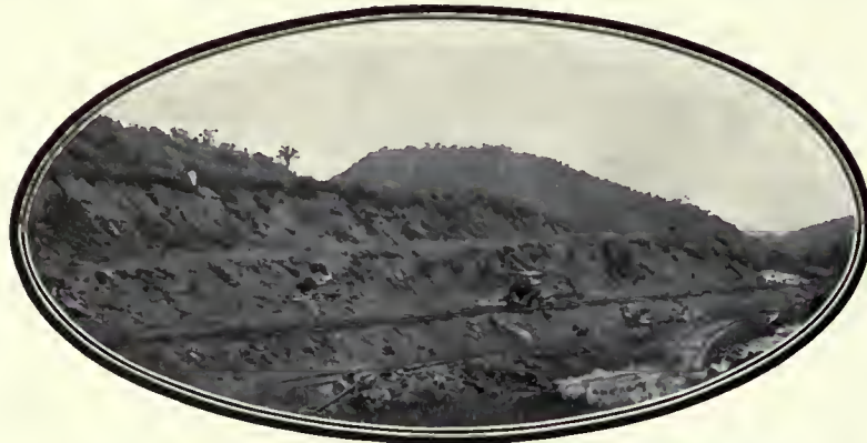
Where the two men are standing was the bottom level in Culebra Cut which the French company reached. The motor car is on a level sixty-five feet lower which represents the digging done by the United States in this section of Culebra Cut.
