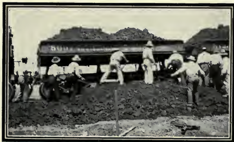
Dumping a Car Load of Spoil.
