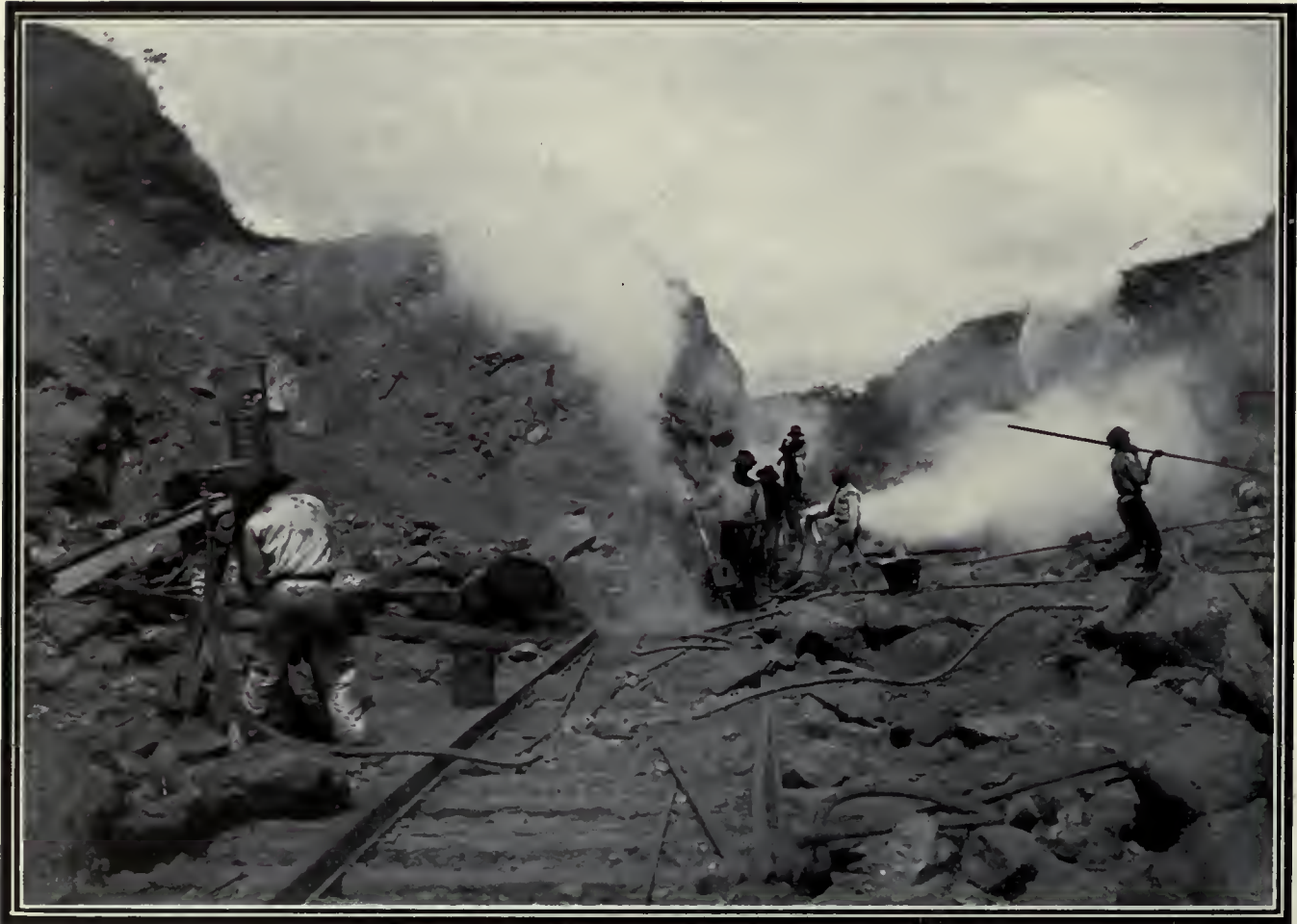
DRILLING FOR THE BLASTS IN CULEBRA CUT
