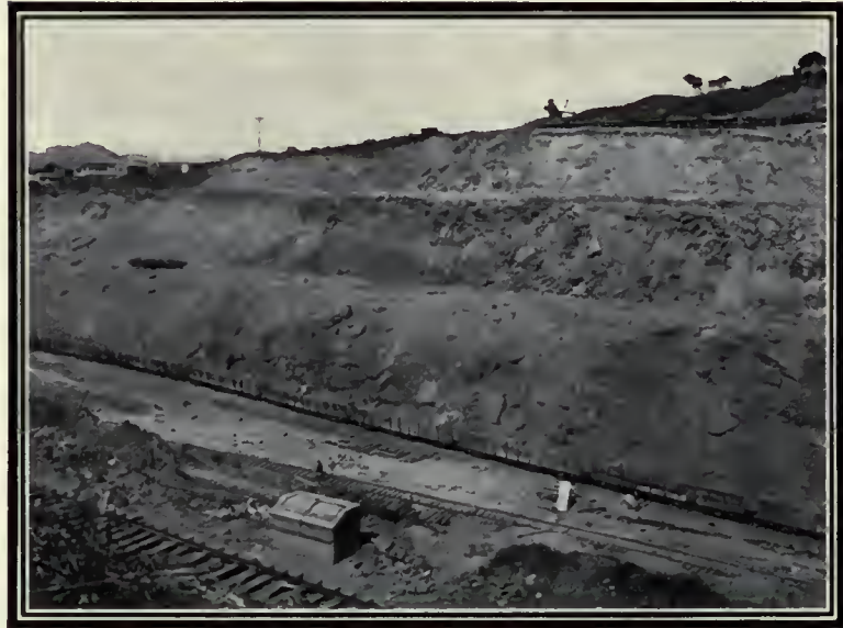
Culebra Cut—The benches or levels by which the excavation is widened. A steam shovel's furrow is forty feet wide.
