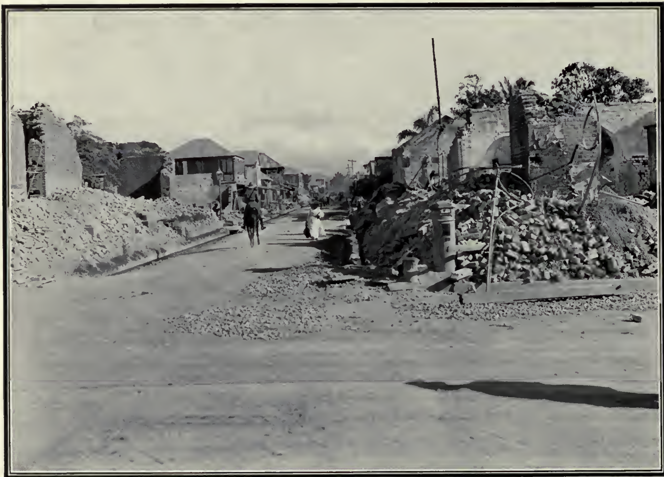
THE BUSINESS CENTER OF KINGSTON A typical scene of the havoc wrought by the earthquake.
