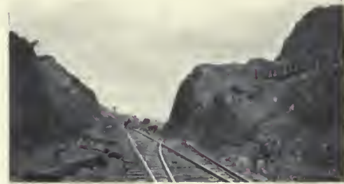
In the Trap Rock — A section of the Canal at Bas Obispo, where the excavation is down to the stratum which must be drilled and blasted.
