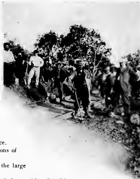
Spanish laborers in Culebra Cut. Mr. Maxwell, of Cincinnati, inspecting them.
