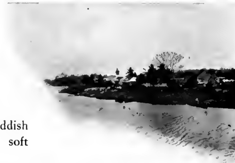
Valley of The Chagres — The old town of Gatun which will be obliterated by the Dam and Lake.
