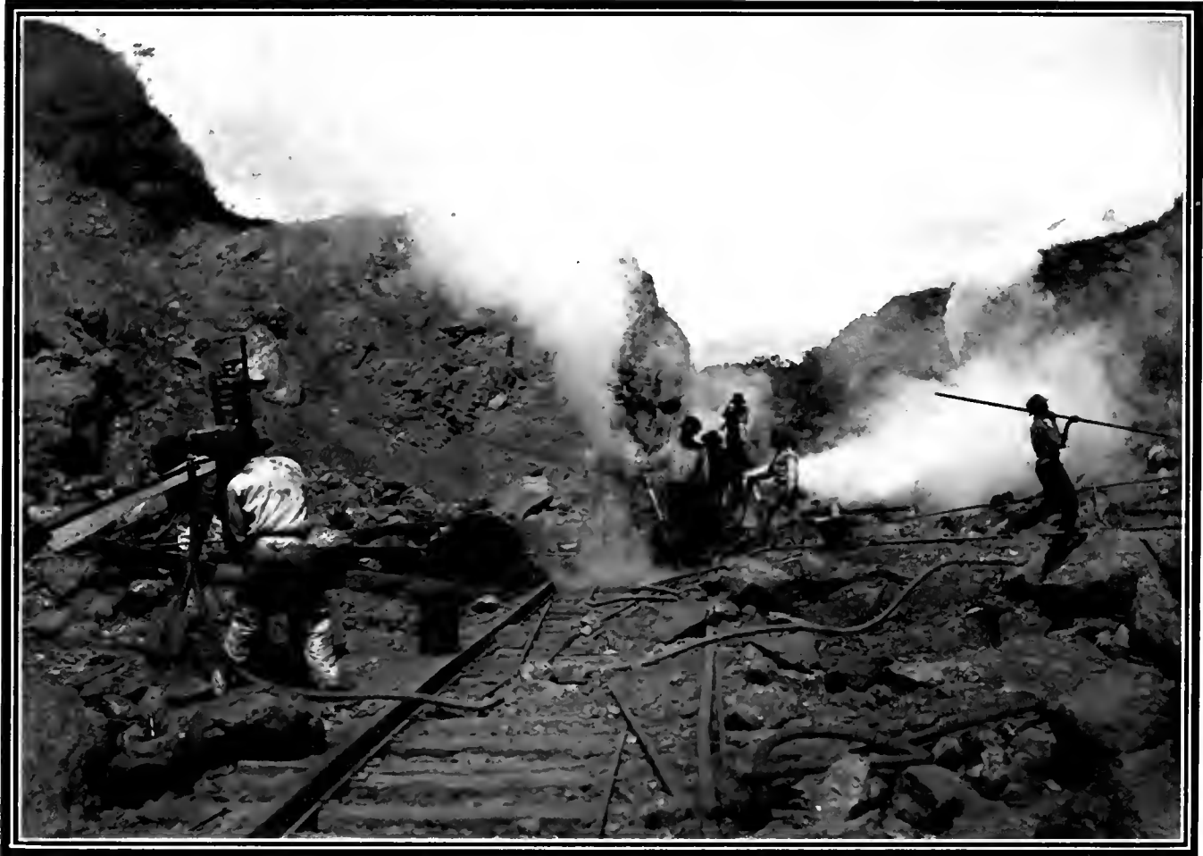
DRILLING FOR THE BLASTS IN CULEBRA CUT
