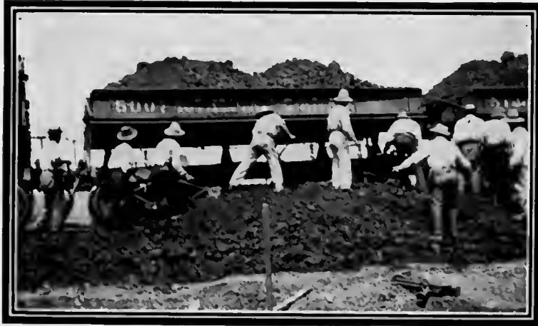
Dumping a Car Load of Spoil.
