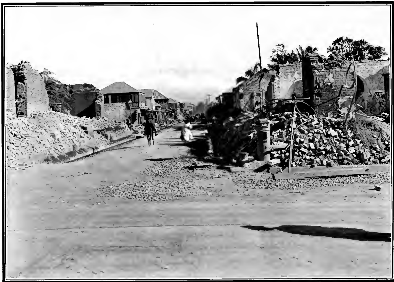
THE BUSINESS CENTER OF KINGSTON A typical scene of the havoc wrought by the earthquake.
