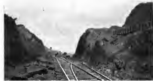
In the Trap Rock — A section of the Canal at Bas Obispo, where the excavation is down to the stratum which must be drilled and blasted.
