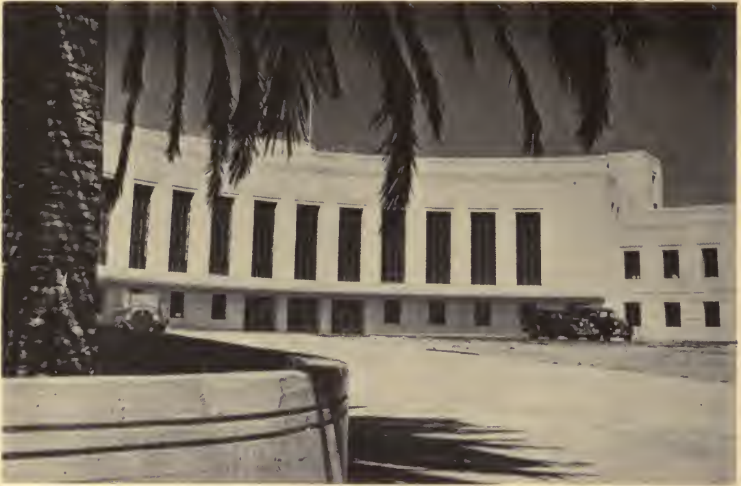
In this horseshoe of concrete Bobby saw what would someday be headquarters for the airport that Treasure Island becomes after the Fair.
