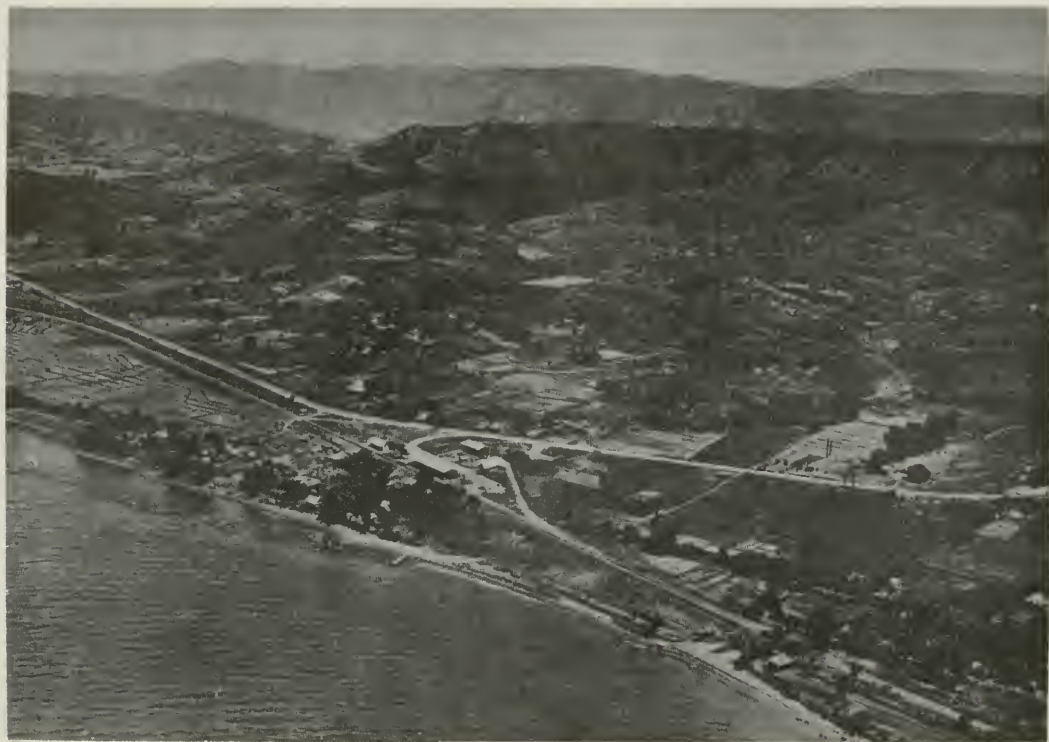
JUNCTION OF COASTAL AND DAMORTIS-ROSARIO ROADS AT DAMORTIS
