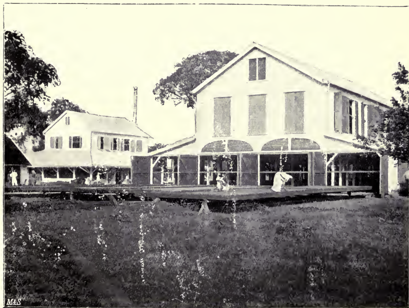
X (b). Cacao drying house in Surinam with moveable platforms to roll out (Original in possession of the Kolonial Wirtschaftliche Komitee, Berlin)
