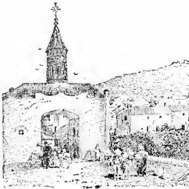
(The gateway to the Bridge of Pines on which Columbus was turned back to discover America.)
