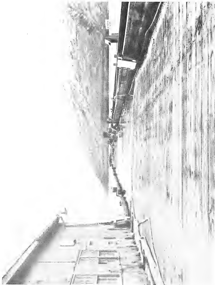
Figure 116 The Fuel Pier at the Naval Station, Kodiak, inundated by Postquake High Tide. (Photograph by U. S. Navy)
