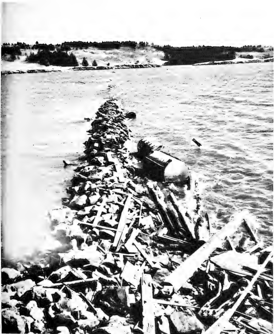
Figure 102 Southwest Breakwater at Kodiak shortly after the Earthquake with some of the battered remains of the King Crab Cannery (Photograph by U. S. Army)
