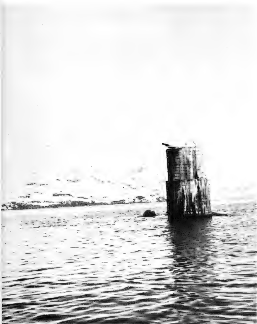
Figure 178 Concrete pylon of the navigation light located at the entrance to Port Valdez (see Figure 177). The light was destroyed by a huge wave that passed southwards out of Valdez Narrows. Steel reinforcing rods at an elevation of about 37 feet above MLLW were bent in the direction of flow. (Photograph by H. Coulter & R. Migliaccio)
