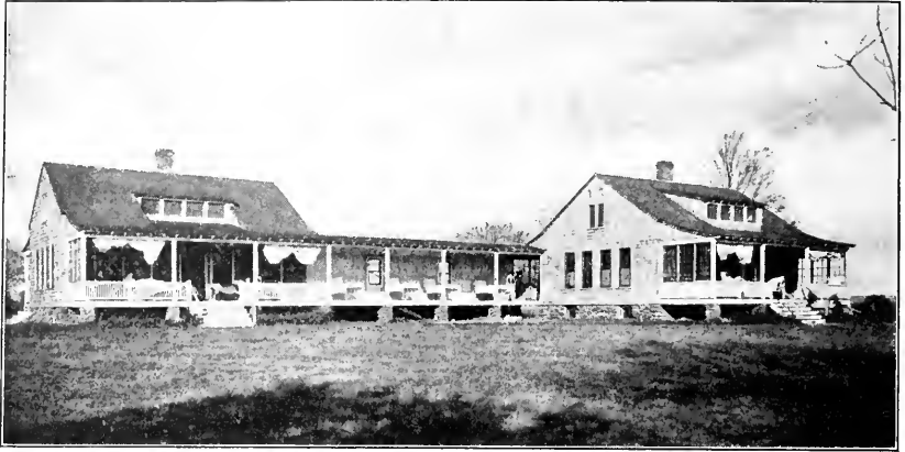
FIG. 157.—OPEN-AIR GALLERY JOINING TWO BUILDINGS. Gaylord Farm Sanatorium, Wallingford, Conn.
