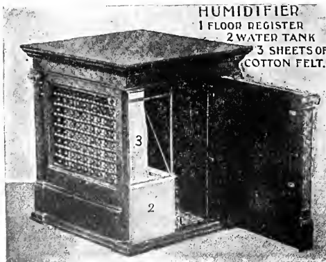
FIG. 41.—HUMIDIFIER FOR HOT-AIR REGISTERS.
