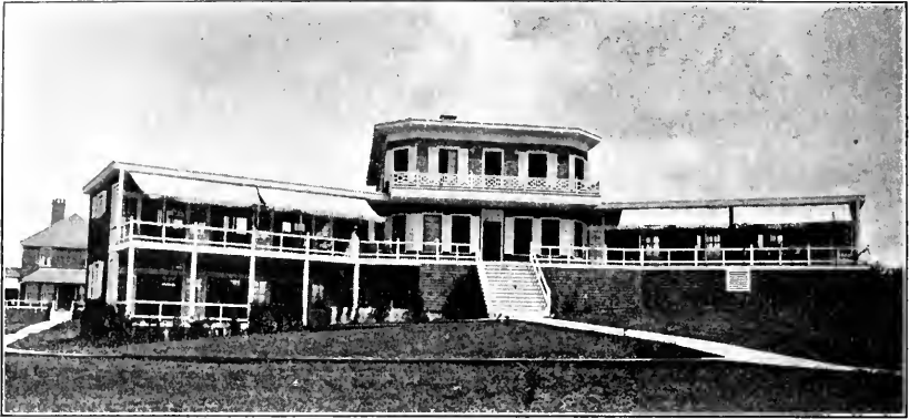
FIG. 163.—OPEN-AIR PAVILION CONNECTED WITH MAIN BUILDING. Infirmary rooms upstairs. Maine State Sanatorium. Designed by Dr. Estes Nichols, Hebron, Me.
