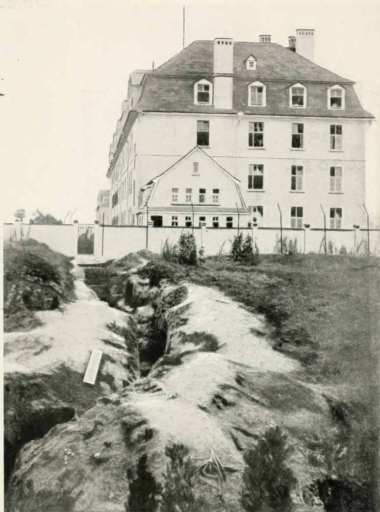
The track of the Holzminden Tunnel after being dug up.
