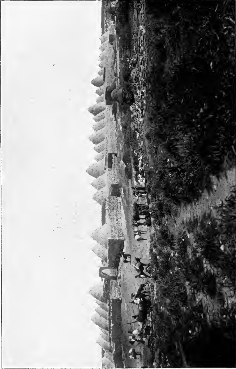
A DOME VILLAGE IN NORTHERN MESOPOTAMIA. On account of the almost entire lack of timber the villagers are compelled to make their roofs by using sun-dried brick or adobe in the form of the dome. In the center of the dome, as a rule, there is a hole which acts both as chimney and as window. These houses are mostly connected by semi-underground passages.
