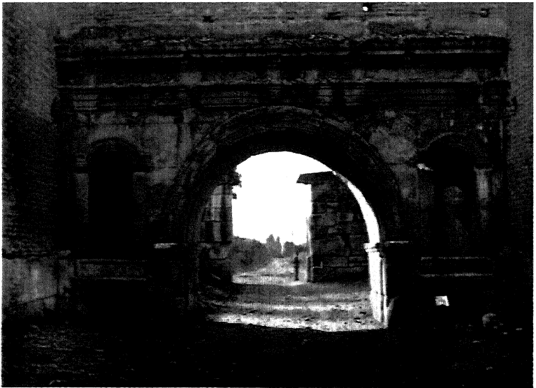
Another of the massive, stone-built Nicean gates.
