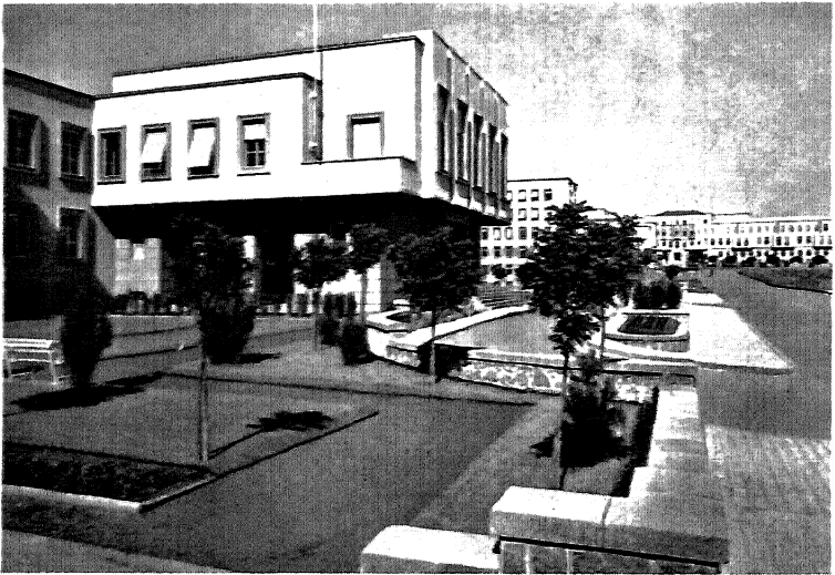
The Ministry of Public Works, Ankara.
