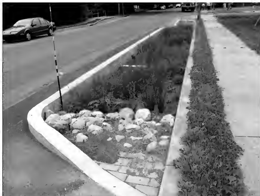
Bio-retention (bump-out) on Locust Street.
