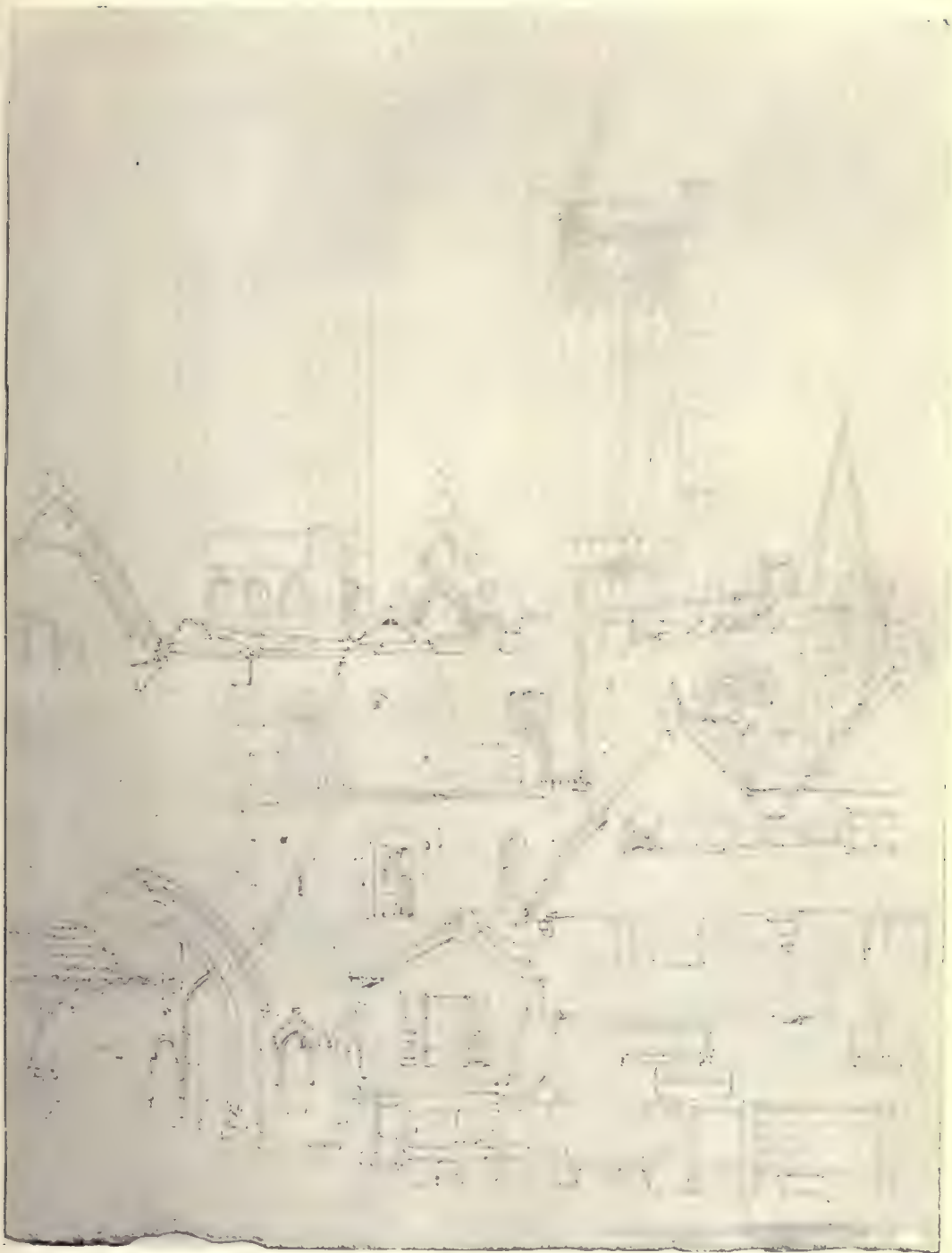
LINCOLN CATHEDRAL, FROM THE SOUTH-WEST
