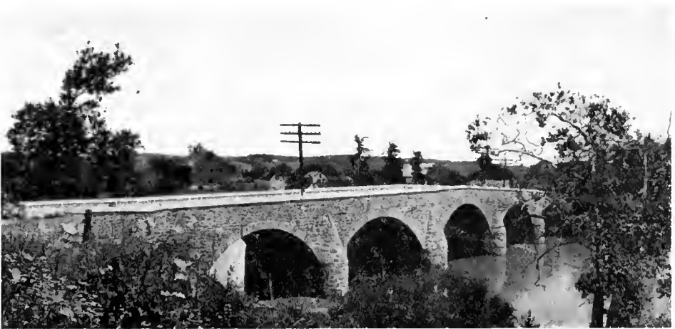
Old Tollhouse Big Conococheague Bridge
