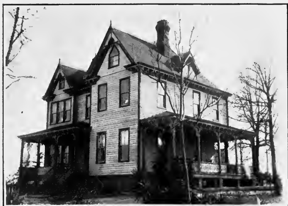
BUILDING NOW USED AS A LIBRARY.
