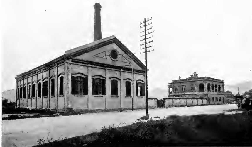
CHINA LIGHT AND POWER COMPANY, LTD.—GENERAL VIEW OF WORKS AT KOWLOON.
