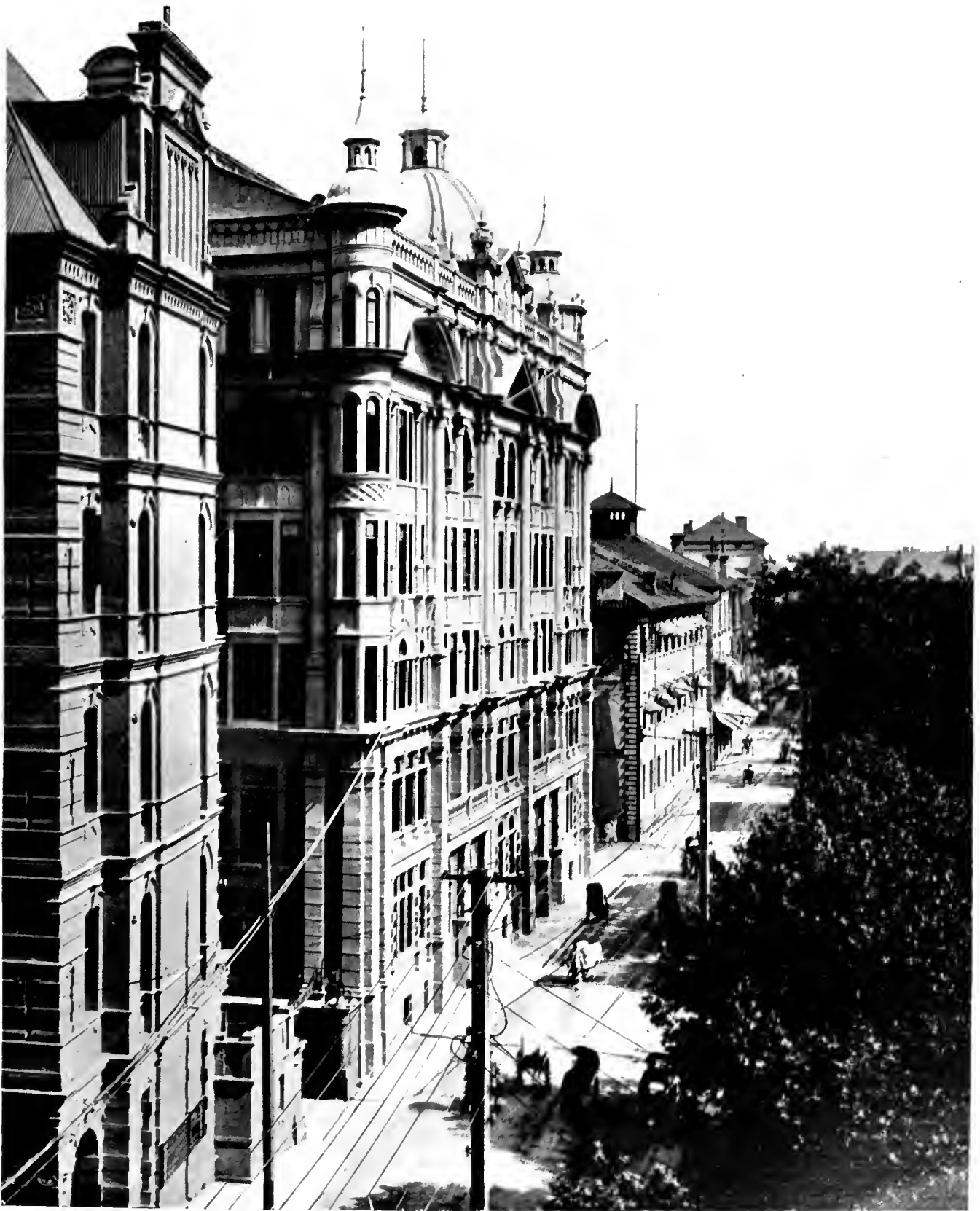
THE SHANGHAI MUTUAL TELEPHONE COMPANY'S NEW PREMISES IN KIANGSE ROAD.
