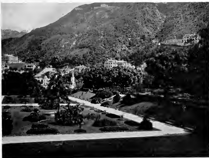
GARDENS, LOWER TERRACE.
