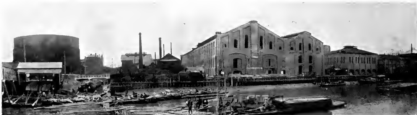
THE GAS WORKS.
