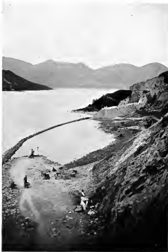
CONSTRUCTION SCENE ON THE KOWLOON-CANTON RAILWAY.
