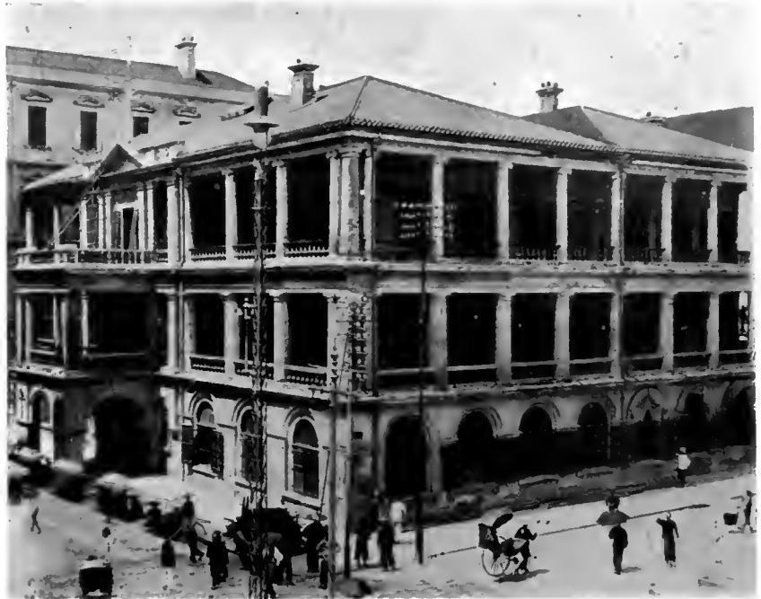
JARDINE, MATHESON & CO.'S OLD PREMISES. (Demolished October, 1907.)
