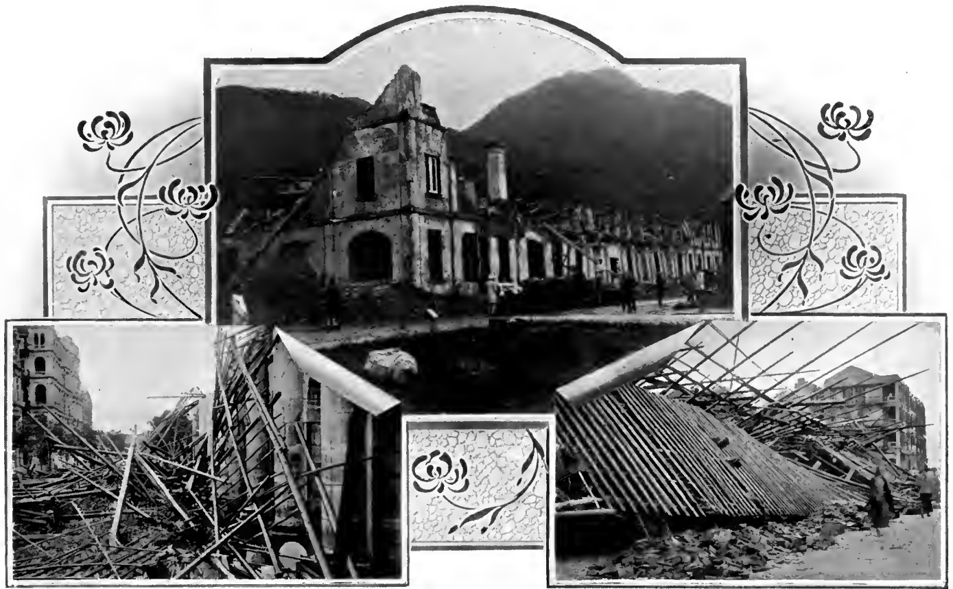
THE GREAT TYPHOON—DAMAGE DONE ON SHORE.
