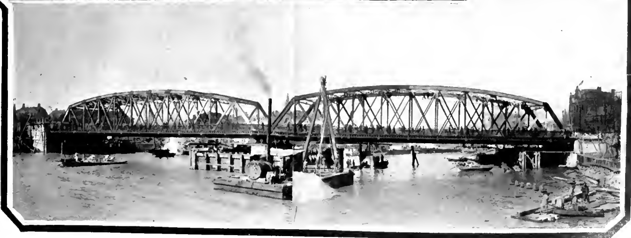
HOWARTH ERSKINE, LTD. THE CHEKIANG ROAD BRIDGE. A CONSTRUCTION SCENE. THE GARDEN BRIDGE.
