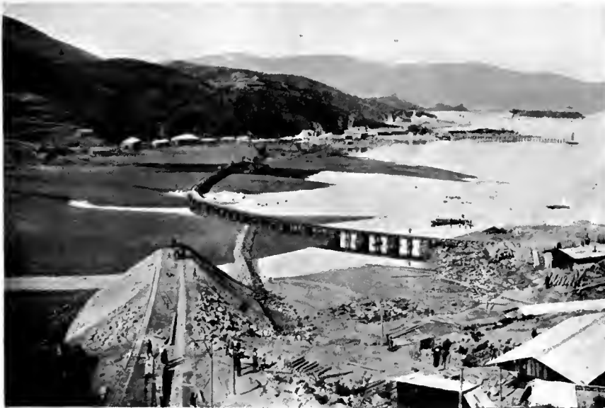
CONSTRUCTION SCENE ON THE KOWLOON-CANTON RAILWAY.
