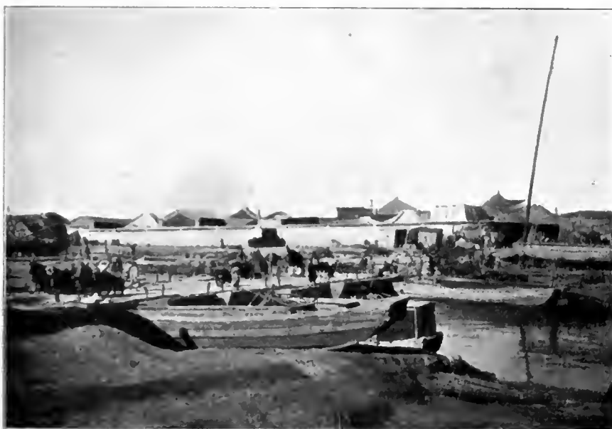
A PONTOON BRIDGE, TIENTSIN.
