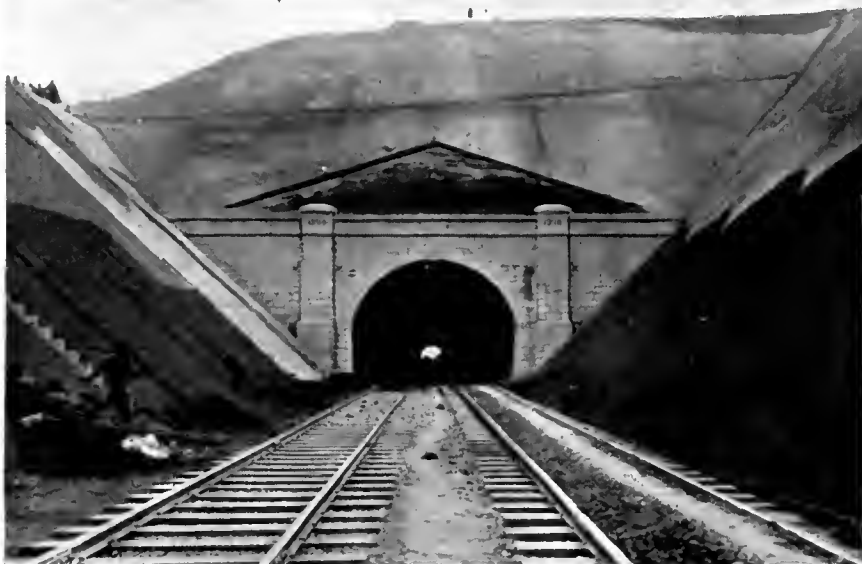
THE CHINKIANG TUNNEL—SHANGHAI-NANKING RAILWAY.
