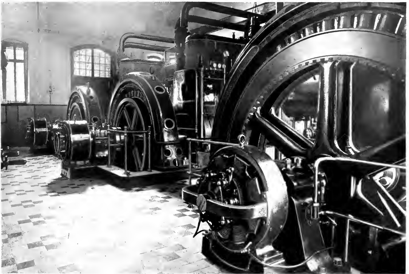
SIEMENS SCHUCKERTWERKE.—THE NATIVE CITY POWER-STATION.
