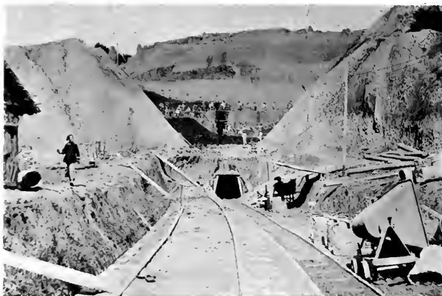
CONSTRUCTION WORK ON THE CHINKIANG TUNNEL—SHANGHAI-NANKING RAILWAY.
