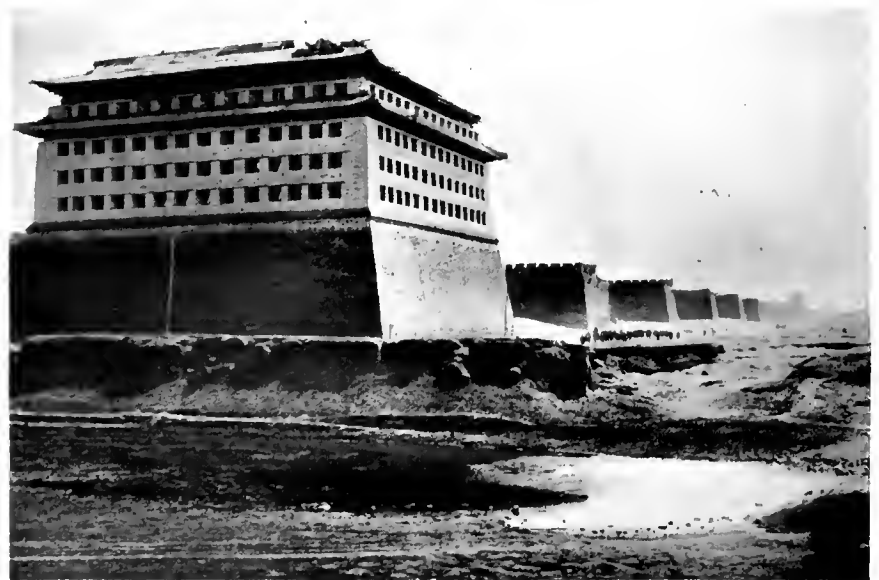
WEST CORNER OF PEKING WALL.
