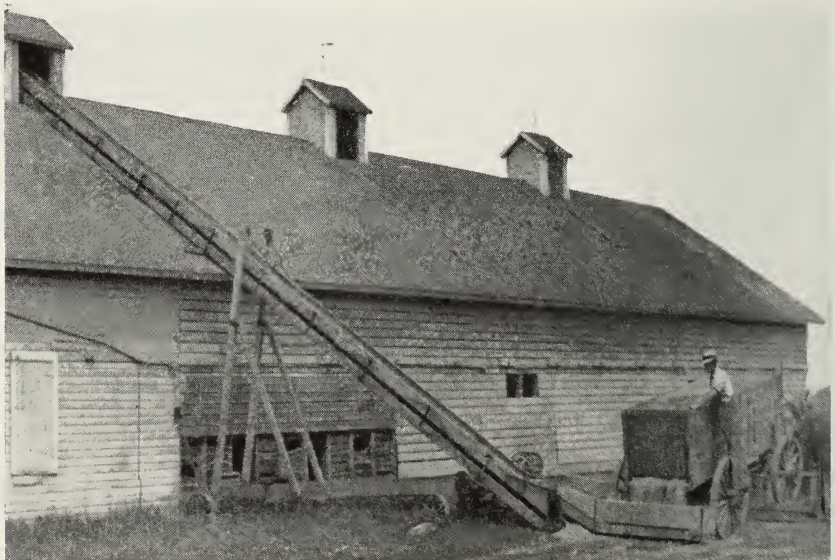
FIG. 17.—ELECTRIC POWER REPLACING HORSE POWER FOR ELEVATING GRAIN
