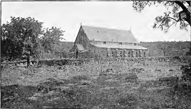
THE NEW CHURCH.
