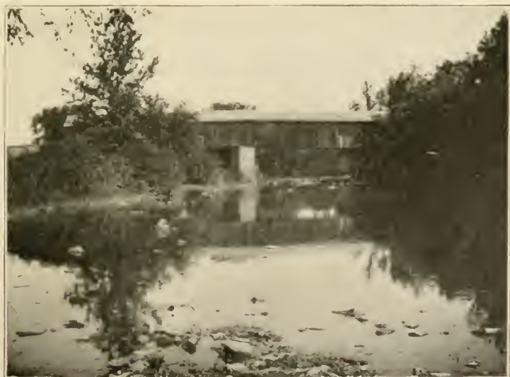
SPRING GARDEN BRIDGE
