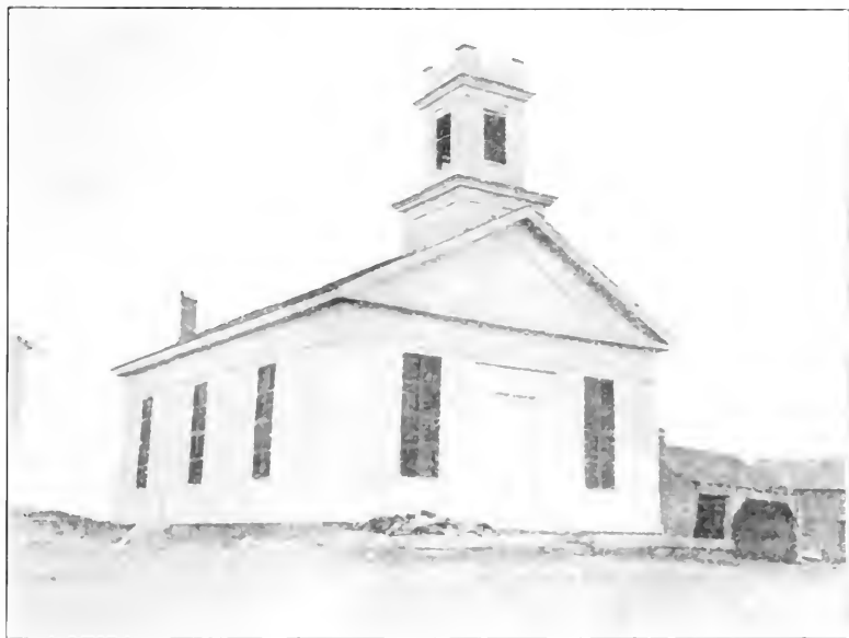
TOLLAND, MASS. CONGREGATIONAL CHURCH AS IT APPEARS 1905. (EFFECTED 1-41)
