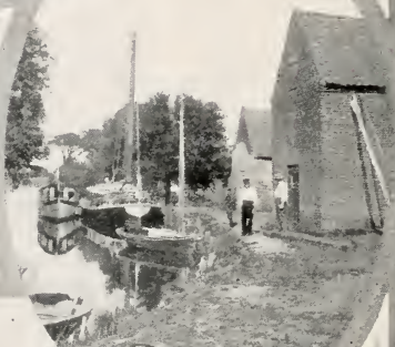
BROADS SOUTH WALSHAM STAITHE
