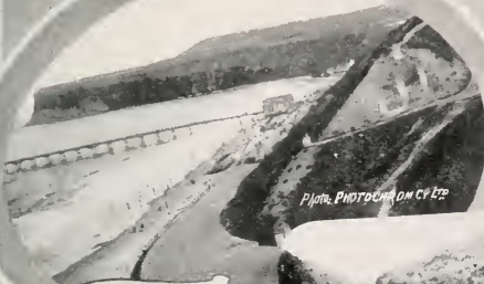
SALTBURN, HUNTCLIFFE & PIER.
