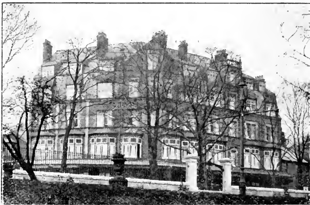
SPA HYDRO FROM KURSAAL GARDENS.
