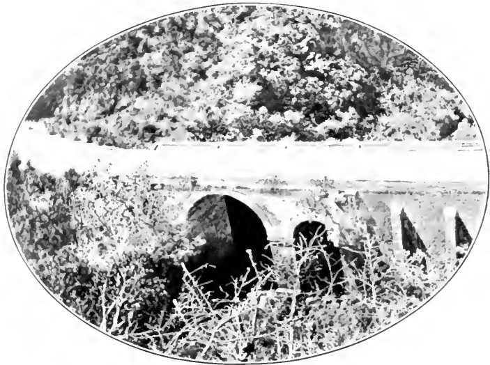
OLD SPANISH BRIDGE
