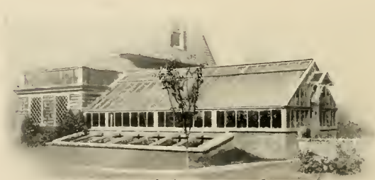
Heated Frames attached to the Greenhouse. — These frames have bricked up sides. At time of taking photo (Oct. 20), was used as a hot bed and filled with lettuce. Later on heat is supplied from the greenhouse boiler by hot water pipes around the frame, carrying them right through the winter. This snug arrangement of frames, greenhouse and stable, is owned by A. J. Morgan, of Larchmont, N. Y. For section detail of these masonry frames see page 9.
