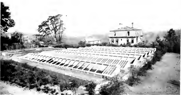
Made deeper than usual, filling the triple use of hot beds, cold and storage frames. These are at Forest Hill Cemetery, Mass.
