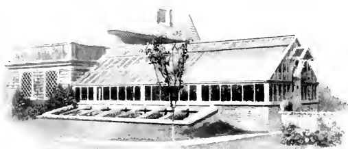
Heated Frames attached to the Greenhouse. — These frames have bricked up sides. At time of taking photo (Oct. 20), was used as a hot bed and filled with lettuce. Later on heat is supplied from the greenhouse boiler by hot water pipes around the frame, carrying them right through the winter. This snug arrangement of frames, greenhouse and stable, is owned by A. J. Morgan, of Larchmont, N. Y. For section detail of these masonry frames see page 9.
