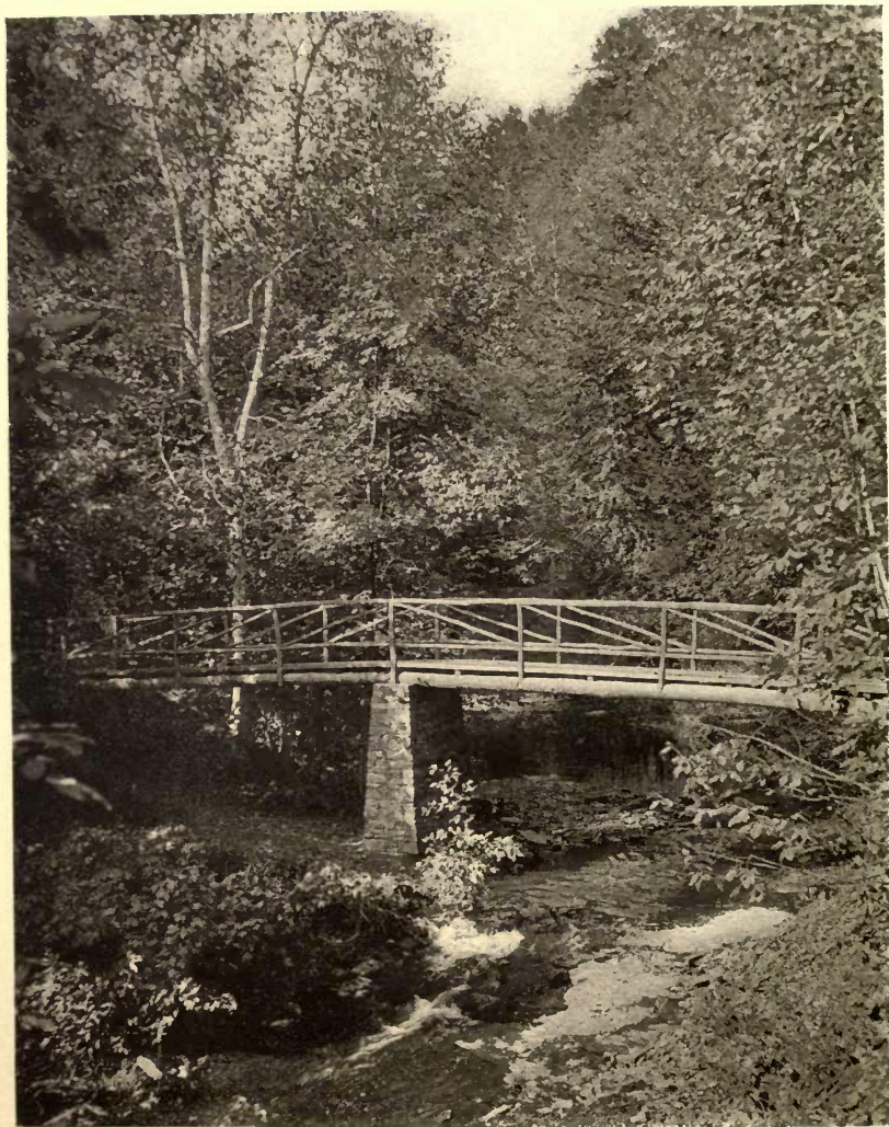
FOOT-BRIDGE AT RENNELAERVILLE, N.Y.
