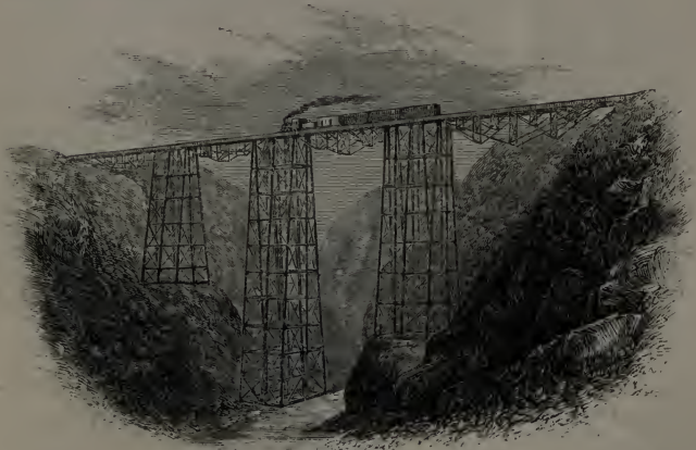
RAILWAY BRIDGE OVER VERRUGAS RIVER.
