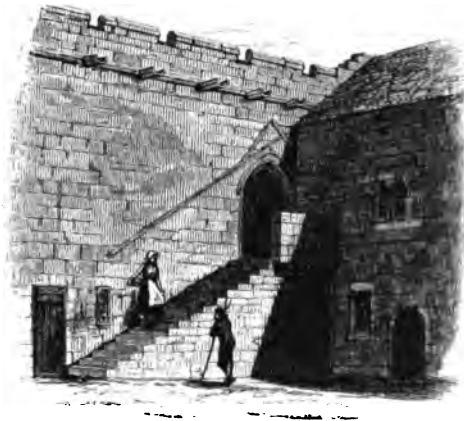
EXTERNAL STAIRCASE—AYDON CASTLE.
