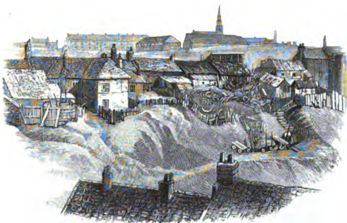
OLD HOUSES NEAR NEWCASTLE.
