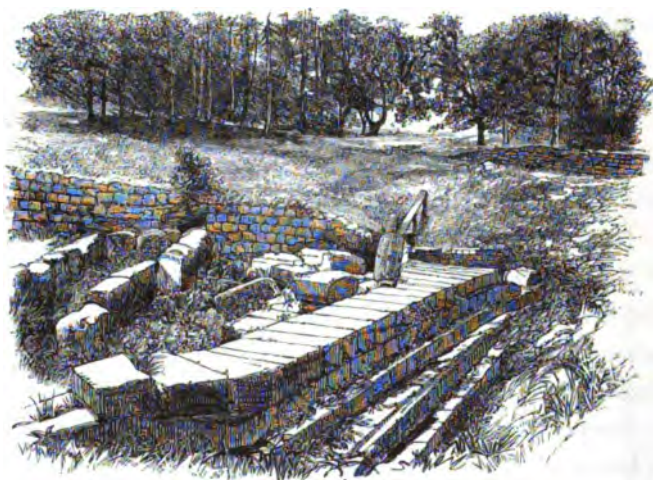
ROMAN BRIDGE. EASTERN ABUTMENT.
