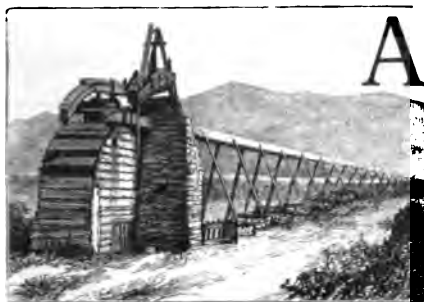
OLD MINE PUMP.
