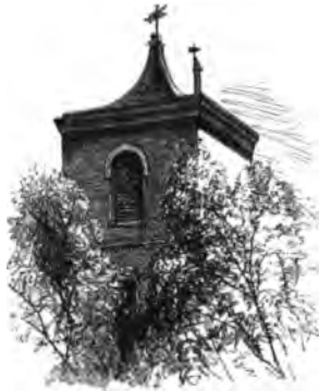
HAYDON CHURCH TOWER.
