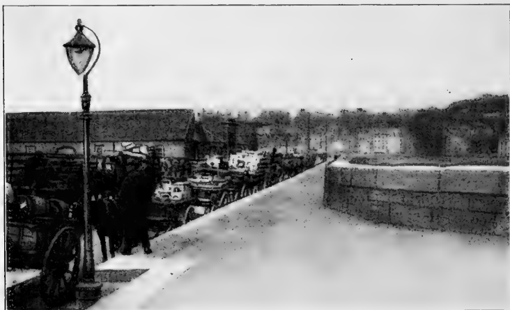
FIG. 165. A view on the dock at St. Peter Port, Guernsey. This shows a line of vehicles awaiting turn unloading fruits and vegetables on the steamer for England. From photograph by the author
