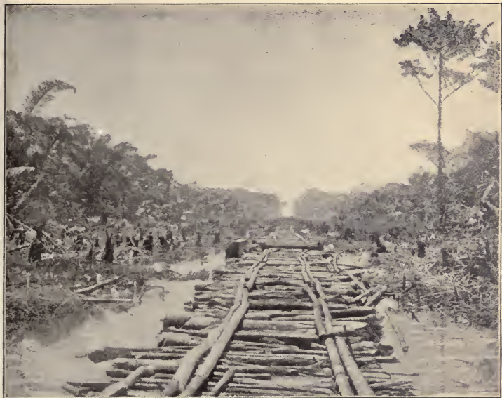
BUILDING RAILROAD THROUGH SWAMP, CORDUROY WITH TIES AND RAILS LAID IN THE BACKGROUND
