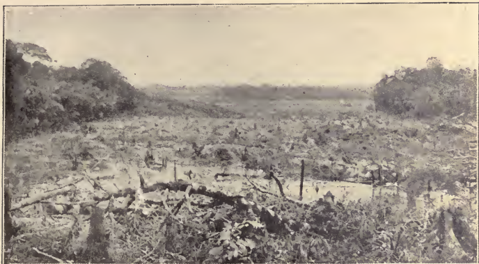
CANAL CLEARING, LOOKING ACROSS LAGUNA BENARD
