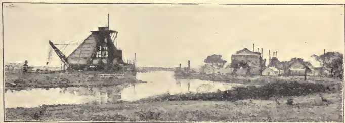
-LA FE, AND DREDGE "CITY OF NEW YORK," LOOKING EASTWARD
