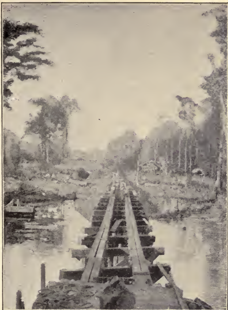
RAILROAD BRIDGE ACROSS BENARD CREEK
