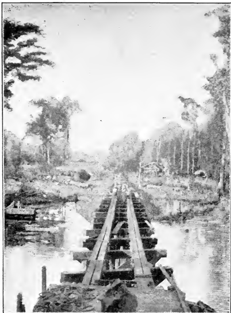
RAILROAD BRIDGE ACROSS BENARD CREEK
