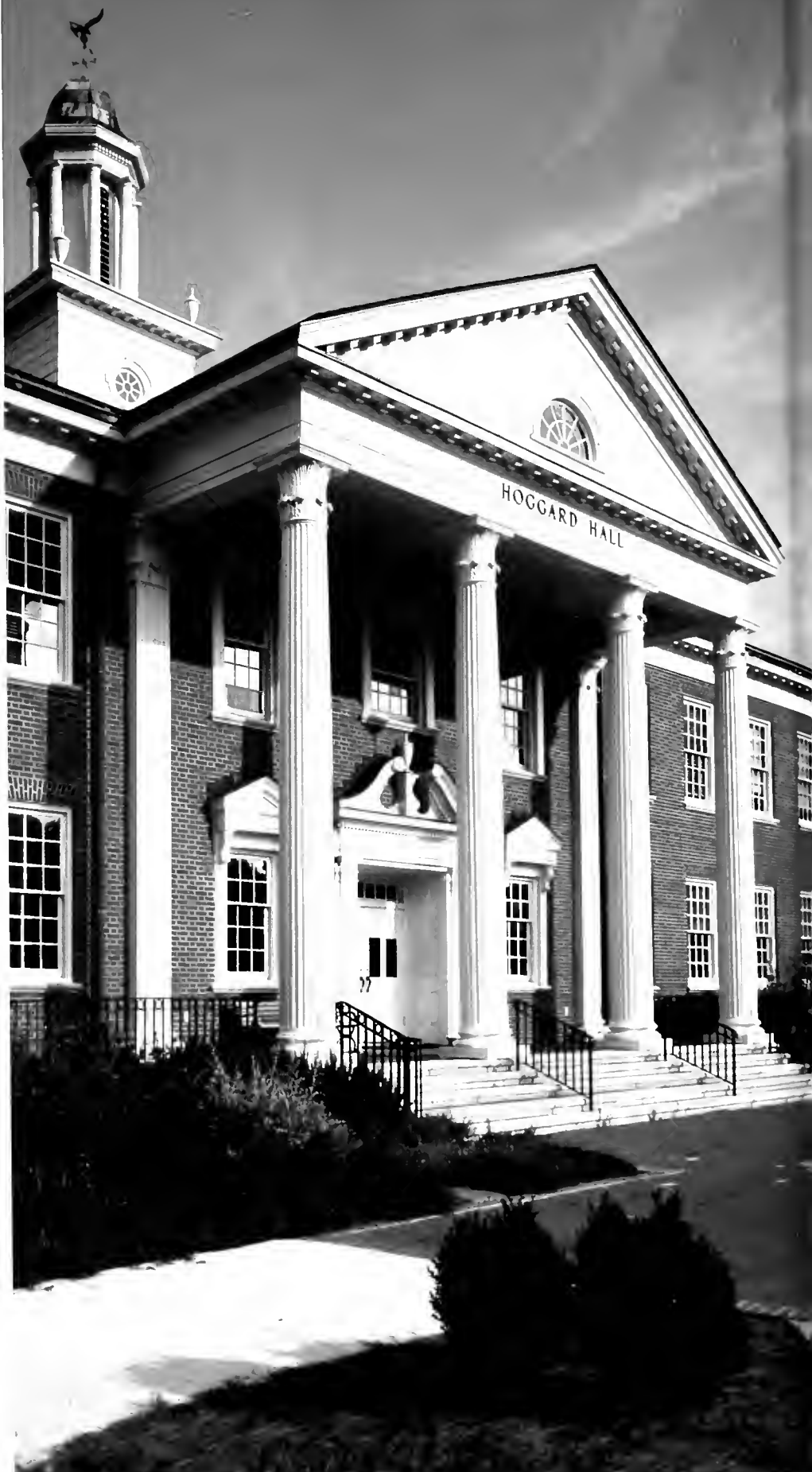
With its Greek Corinthian columns and Flemish bond masonry, Hoggard Hall, one of the three original buildings on campus, exemplifies the modified Georgian architectural style that defines the UNC Wilmington campus. (See story on page 16.)
