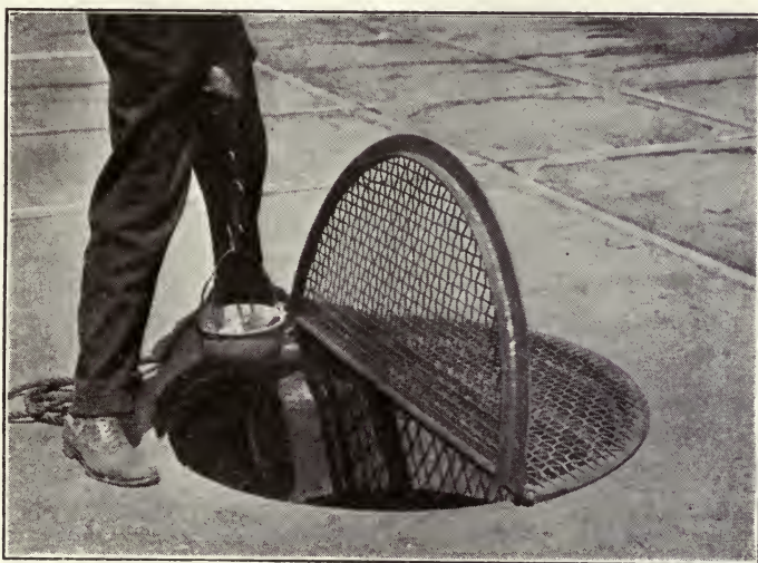
FIG. 105.—Manhole grating.
