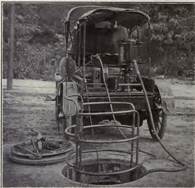
FIG. 86.—Joint-filling apparatus mounted on electric vehicle.
