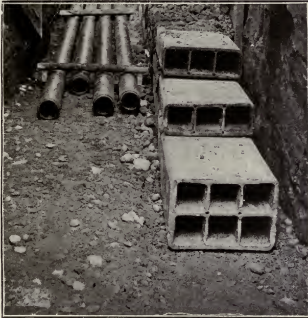
FIG. 20.—Installation of fiber and multiple duct.
