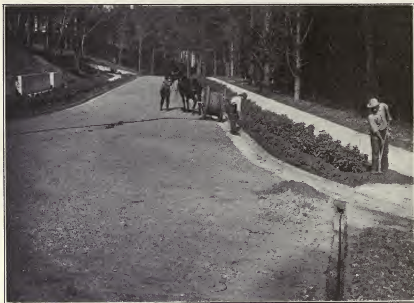
FIG. 50.—Installation of armored cable.
