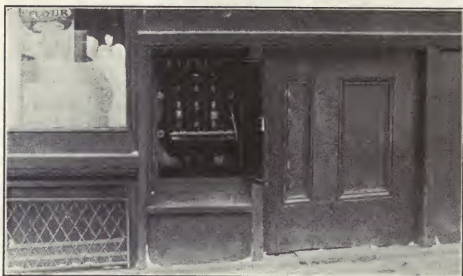
FIG. 47.—Method of installing service box in buildings.
