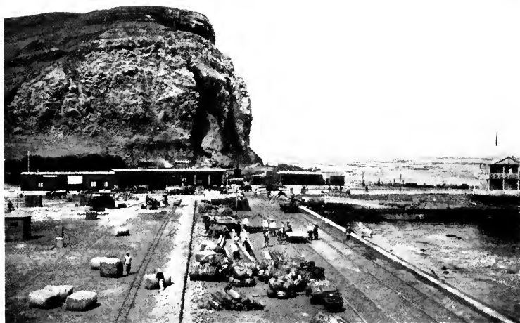
ARICA—THE TERMINUS OF THE NEW CHILEAN RAILROAD FROM LA PAZ
