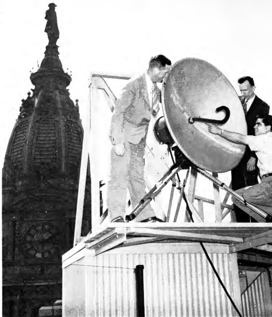
A parabolic reflector, popularly called a "dish," is used to reflect television's microwaves in much the same way that a searchlight projects a beam. The microwave transmitter is contained in a weather-proof cylinder attached to the back of the parabola.
