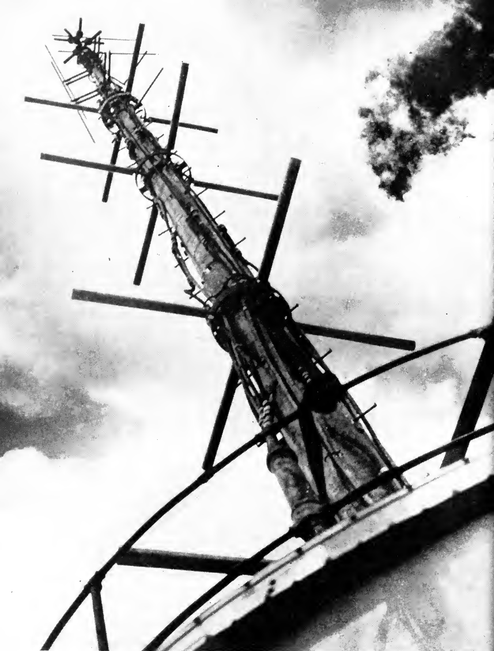
Television antenna of the NBC station, WNBT, atop the Empire State Building, is 1,300 feet above the sidewalks of New York.
