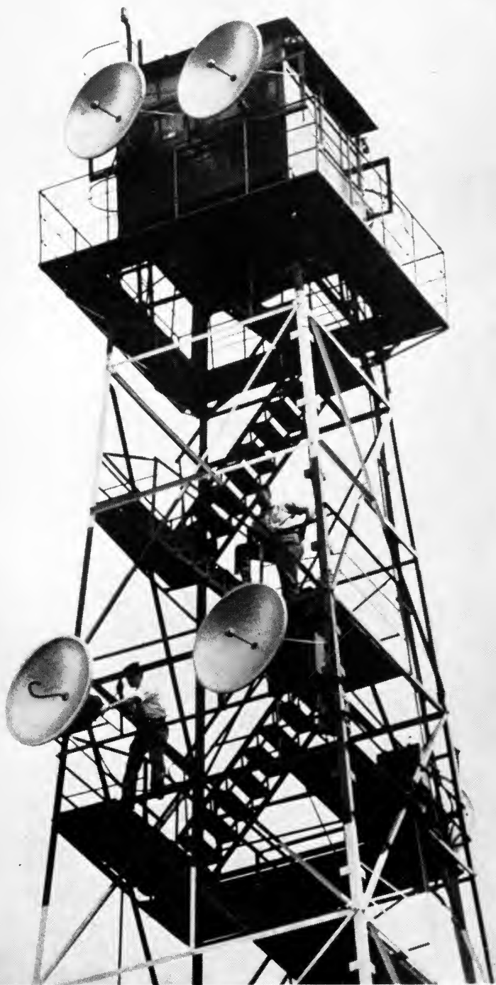
Radio relay stations with 10-foot "dish" reflectors on both sides pick up the television programs and automatically relay them to another relay station or to the main transmitter if it is within range.
