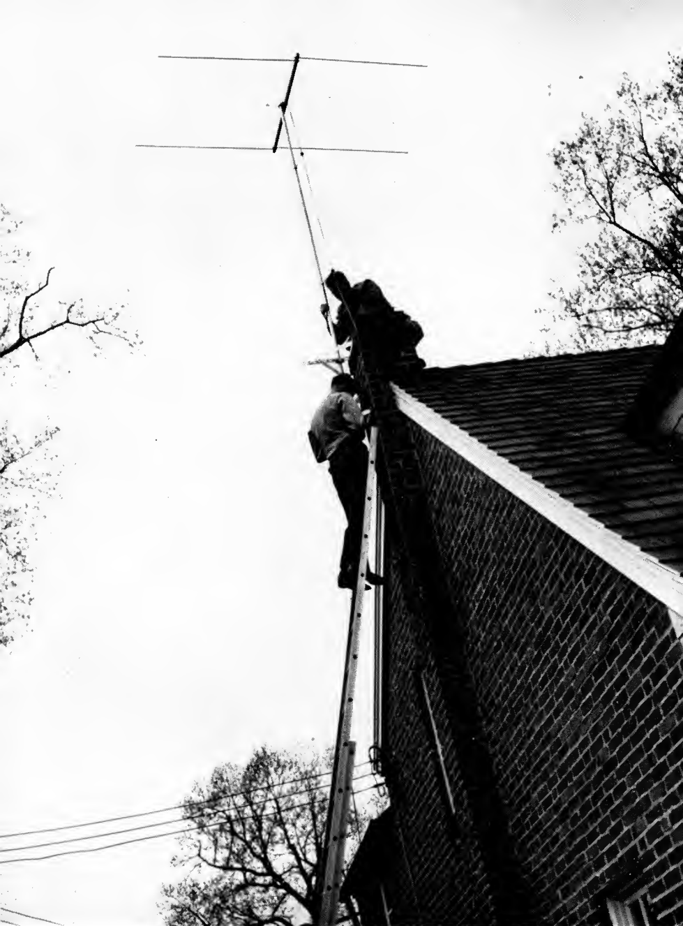
Dipole television antenna with reflector rod.
