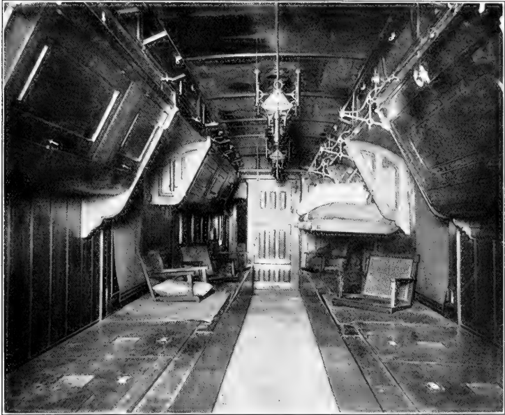
INTERIOR VIEW OF FISH TRANSPORTATION CAR
