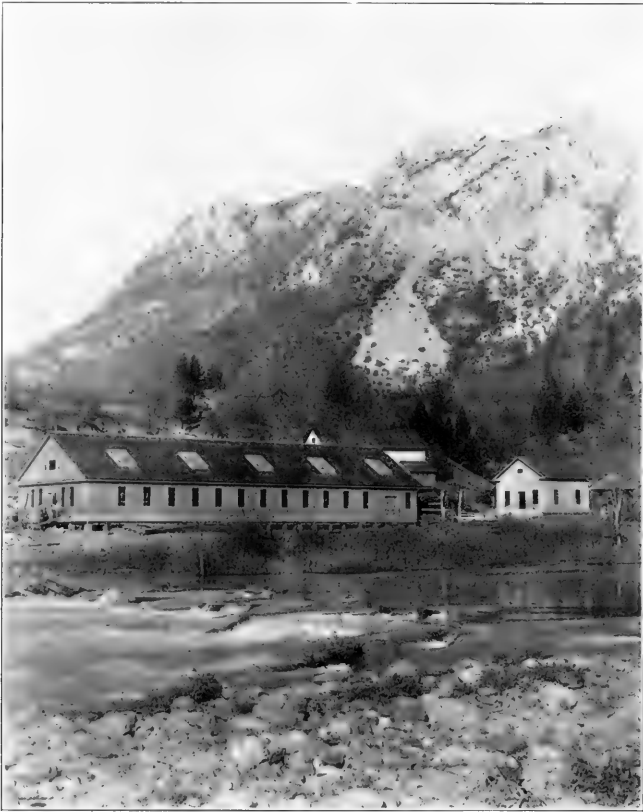
SALMON HATCHERY AT BAIRD, CALIFORNIA
