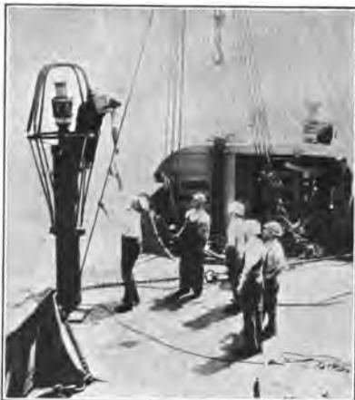
Testing pressure in gas buoy, New York Bay.
