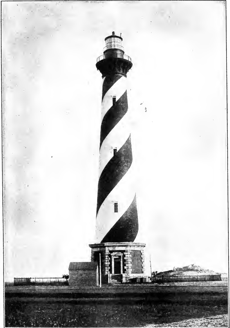
Cape Hatteras Light Station, N. C.
