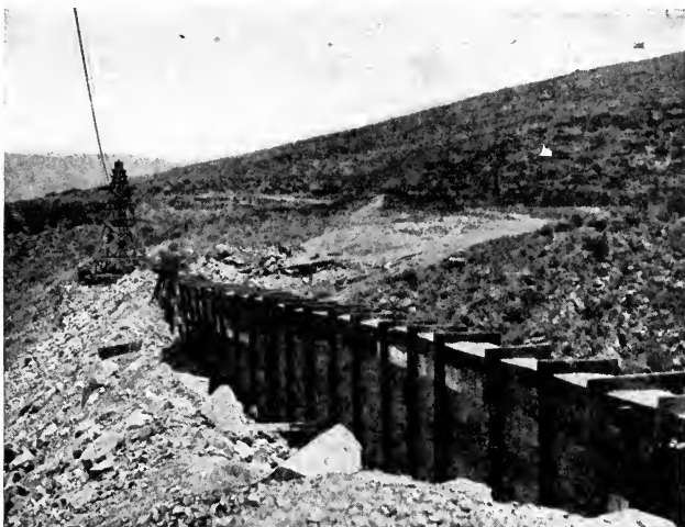
A. LOWER OTAY DAM, CALIFORNIA, SHOWING METHOD OF PROTECTING STEEL PLATES.
