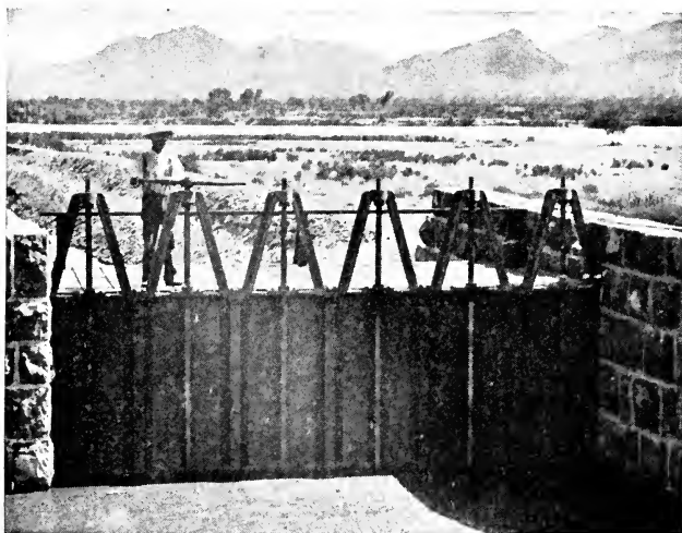
A. MASONRY HEAD-GATES OF CANAL.
