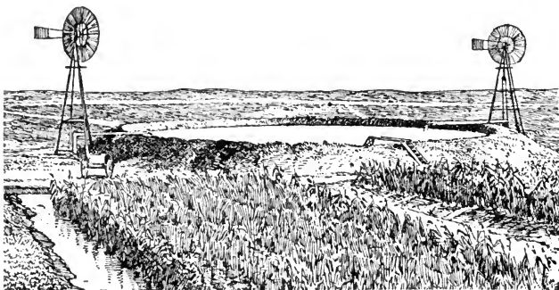
FIG. 87.— Windmill pumping into earth reservoir.
