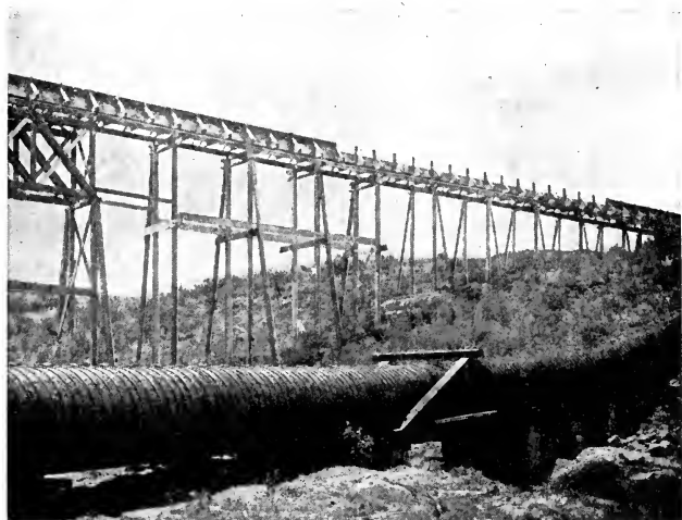
B. OLD FLUME AND REDWOOD PIPE REPLACING IT, REDLANDS CANAL, CALIFORNIA.
