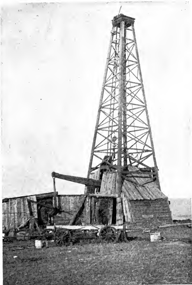
OUTFIT FOR DRILLING DEEP ARTESIAN WELLS.
