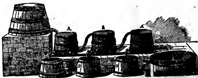
Fig. 56.—LIXIVIATING TUBS, MONNIER'S PROCESS.
