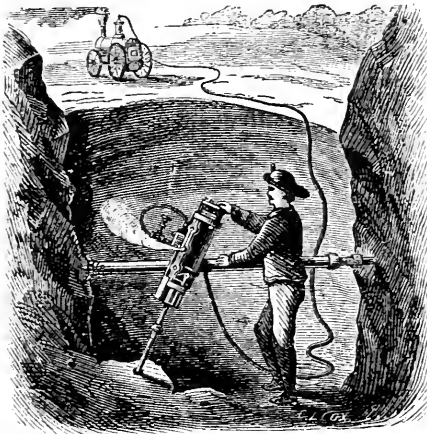
VIEW OF DRILL ATTACHED TO COLUMN, AS ARRANGED FOR USE IN SHAFTS.
