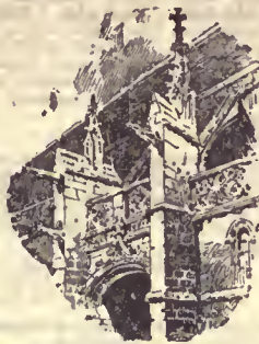
FLYING BUTTRESSES (ST. OULLES, CANN.)
