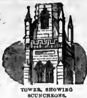
TOWER, SHOWING SCUNCHEONS.
