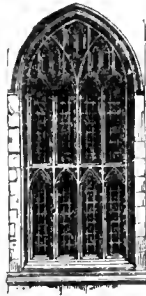
PERPENDICULAR WINDOW WITH TRANSON.
