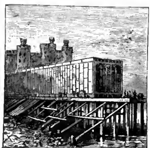
CONWAY TUBULAR BRIDGE IN PROCESS OF CONSTRUCTION.
