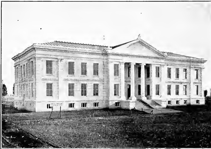
THE COMPLETED COLLEGE OF HISTORY.
