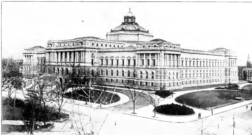
THE LIBRARY OF CONGRESS—WEST AND SOUTH FRONTS.
