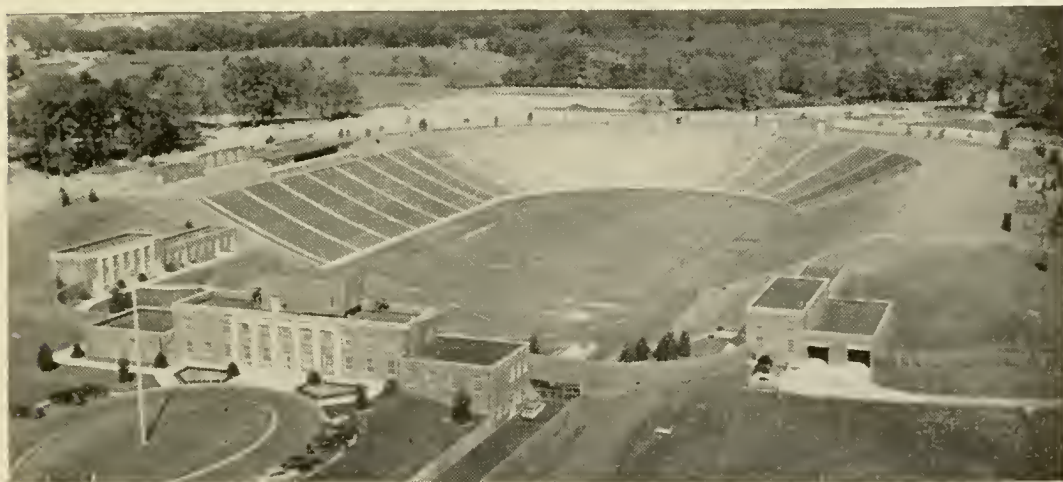
BYRD STADIUM HOME OF THE TERRAPINS Capacity: 35,000
