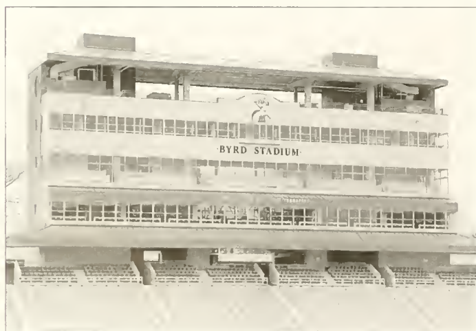
Tyser Tower, shown here from the front, features a spacious press box and a hospitality suite with theater-style seating.
