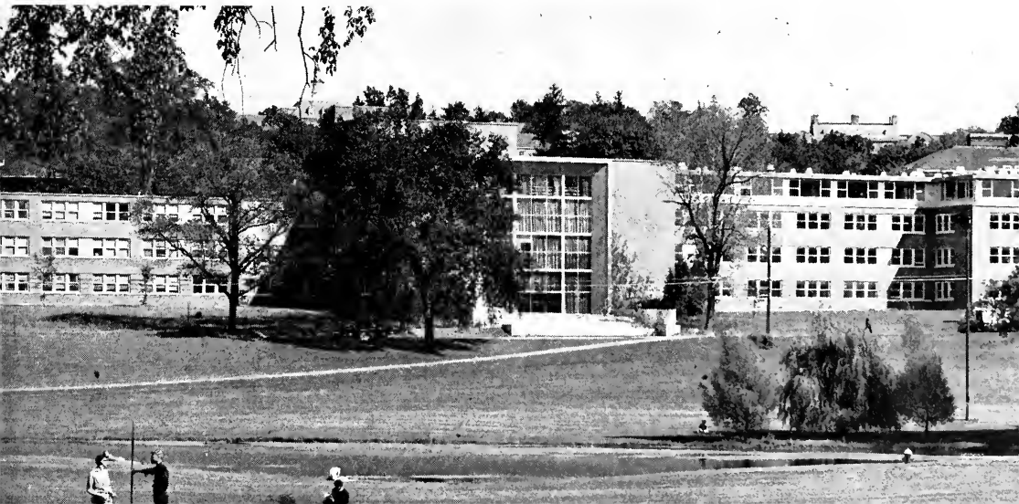
The Justin Morrill Science Center — three of its four sections complete in 1962.
