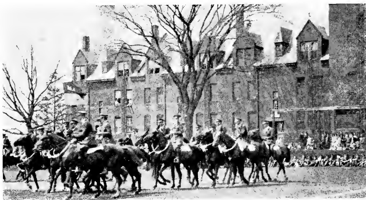
Mounted drill in the 1920's.
