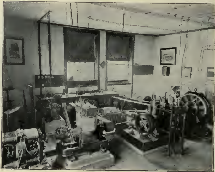
Electrical Engineering—Dynamo Room.
