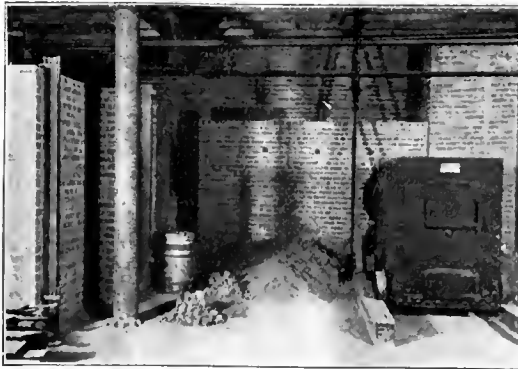
The Furnace Room.
