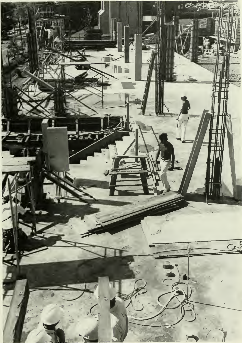
Construction of Dodds Hall begins in 1981.
