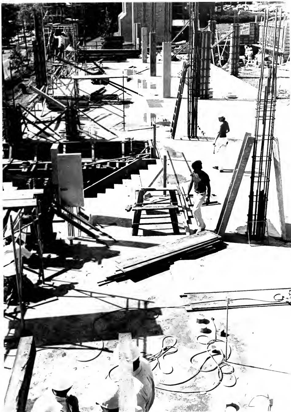
Construction of Dodds Hall begins in 1981.
